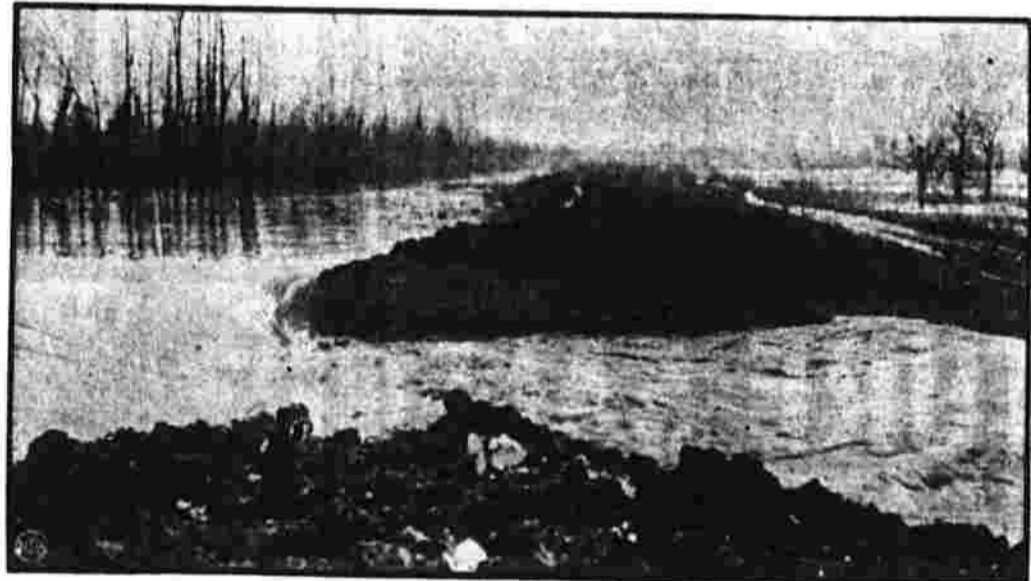
Pent-up waters of the Mississippi rushed through the dynamited gap in the levee with terrific force, flooding farm lands and homes and lapping viciously at the heads of desolated farmers in the 130,000-acre fertile district who looked to it to feed the millions of years gone with the waters. The levee was broken to relieve pressure on the levee and save Cairo, farther downstream, from destruction.
