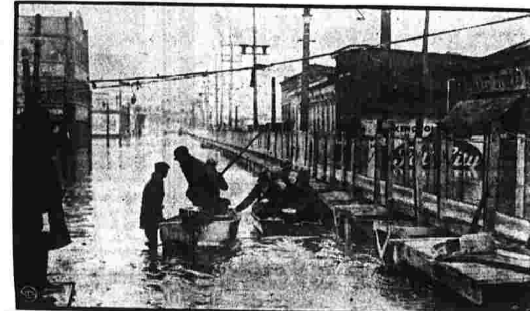
Workers here inspect the almost finished pontoon footbridge which was built in Louisville by a famed whiskey industry built the bridge, for under three planks float oak after oak, made of white tramped over the bridge when it was completed. It was the city's only outlet to the Highlands, the only way—except by boat—to bring in food and medicine for 230,000 homeless.
